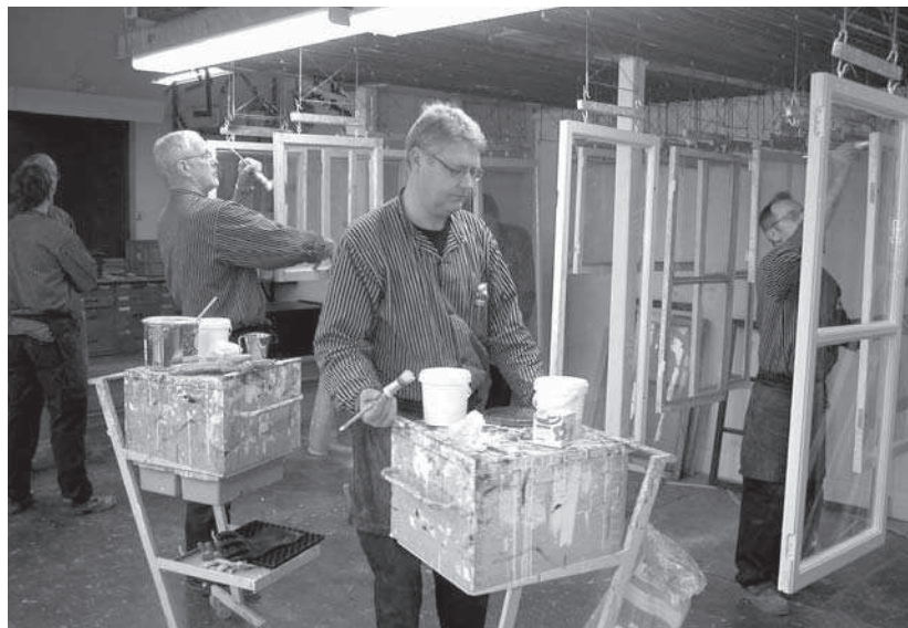
Figure 4 Students at Bjäresjö School, Ystad learning how to use solvent-free linseed-oil paint manufactured by local raw flax material.
