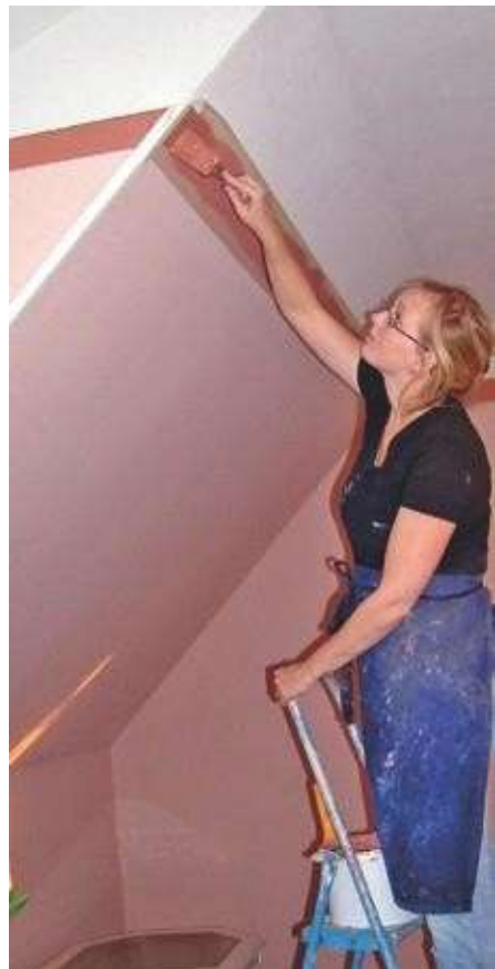
Paint Linus using a Perlon roller or a brush.
