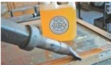
Heat the oil with hot air. Paint immediately.
