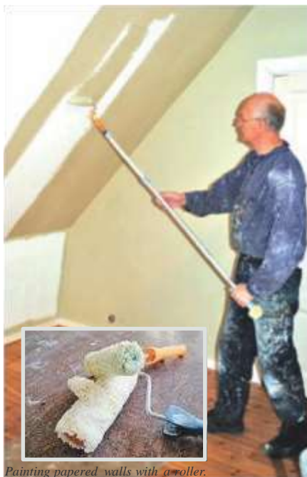
Painting papered walls with a roller.
