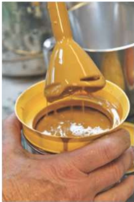
Mix the paint with a hand-held blender.
