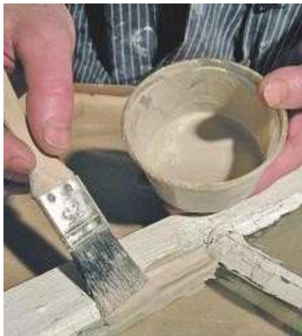
Thinned putty, a simple “delay aging” measure.
